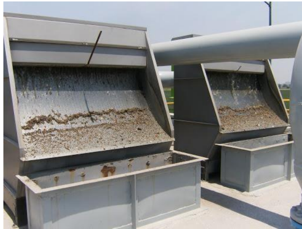
Figure 3. Hydroscreen with speciated rods of 5mm to separate solids from water (JUMAPAC, 2016)
