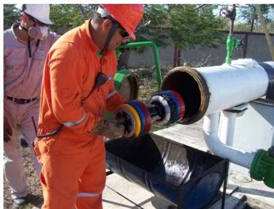
Figure 15 Polly pig used for cleaning pipes 43
