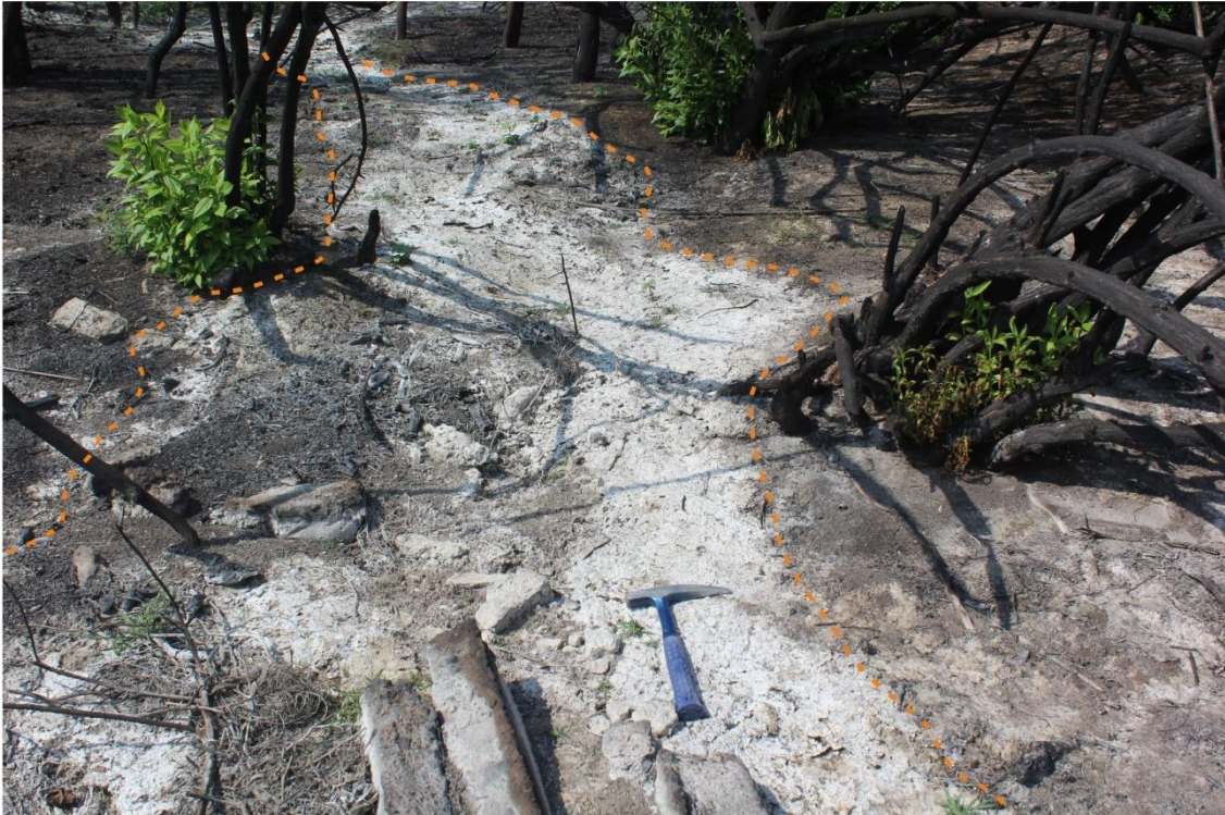
Figure 27. The presence of soluble salt crusts on the surface is due to the capillarity process in areas with saline soils. This process can occur more frequently in dry precipitation due to the evaporation-transpiration of water to the surface. This saline soil is located in Tolas Zone (T17M21P20; see Figure 1B).
