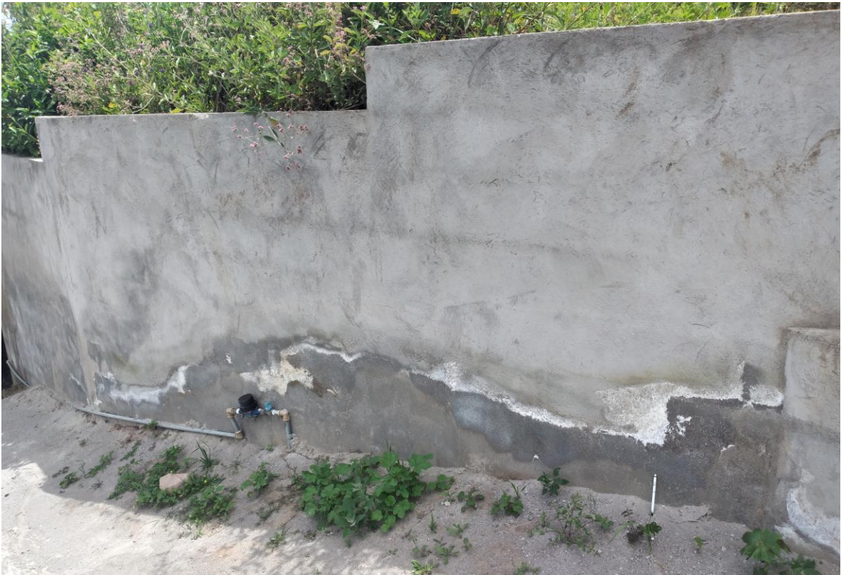
Image 6. The concrete roof presents white spots; the water filtration would cause this.
