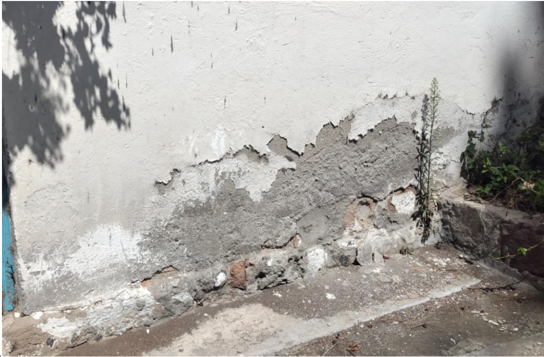
Image 3. Building under weathering agents shows the degradation of building materials.
