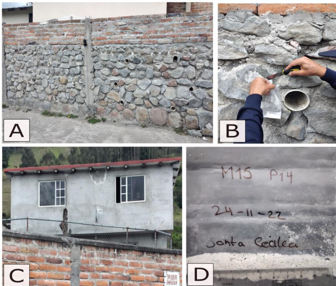
Figure 21. White minerals are present in lava brick walls in Santa Cecilia Community (See location in Figure 1) (A). Collecting crystals from the wall (B). A white splotch on a new house's second floor (C). Sample M15P14 taken (D).
