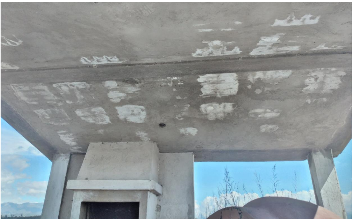
Image 6. The concrete roof presents white spots; the water filtration would cause this.
