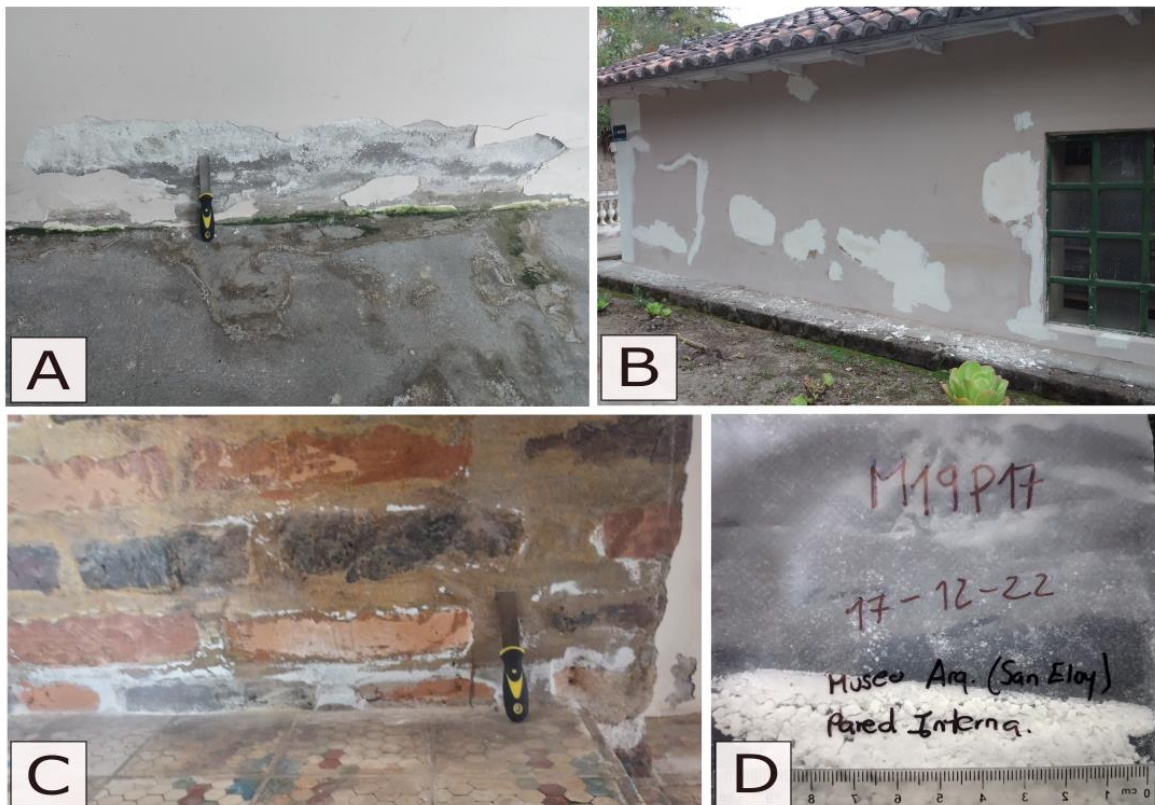
Figure 25. Inner wall with salt crystals in San Eloy (See location on Figure 1) (A). Reparation of the external wall in the Archaeological Museum (B). Clay blocks with salt crystals (C). Sample M19P17 was taken from the analyzed wall.
