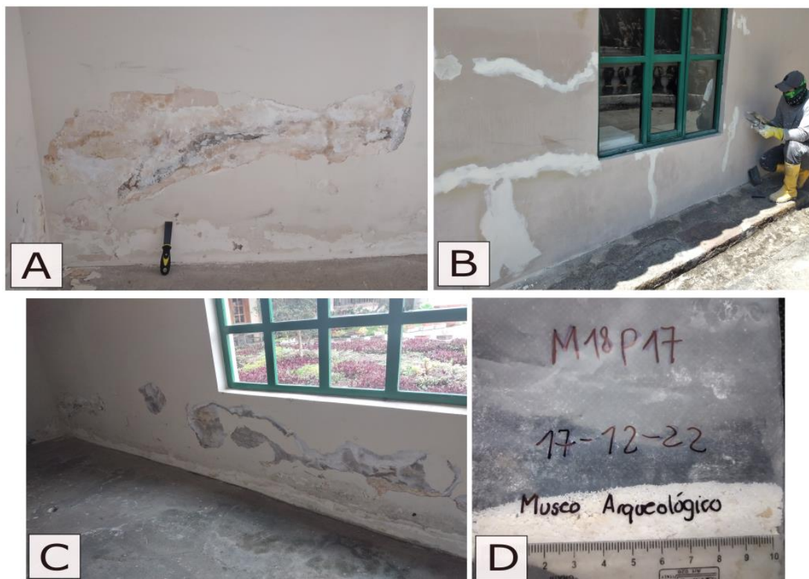
Figure 24. Outer wall with white crystals in San Eloy (See location on Figure 1) (A). Reparation of the wall in the Archaeological Museum (B). Overview of the wall with deterioration (C). A sample M18P17 taken from the external wall (D)
