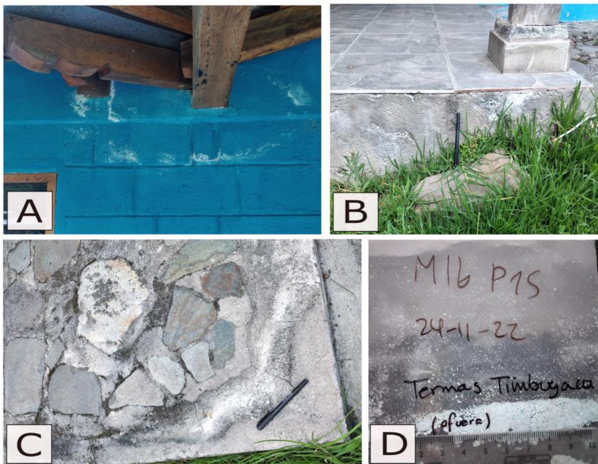
Figure 22. Crystals grow in the upper part of the wall in Timbuyacu Community (See location in Figure 1) (A). White minerals are presented on the floor (B). Crystals develop around volcanic rocks in the soil (C). The sample taken from the walls was analyzed (D).
