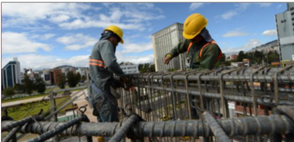
Figure 6. Iron Rods. Iron rods structures employed to enforce slabs and columns. These structures are directly cover by concrete (Adelca, 2020).
