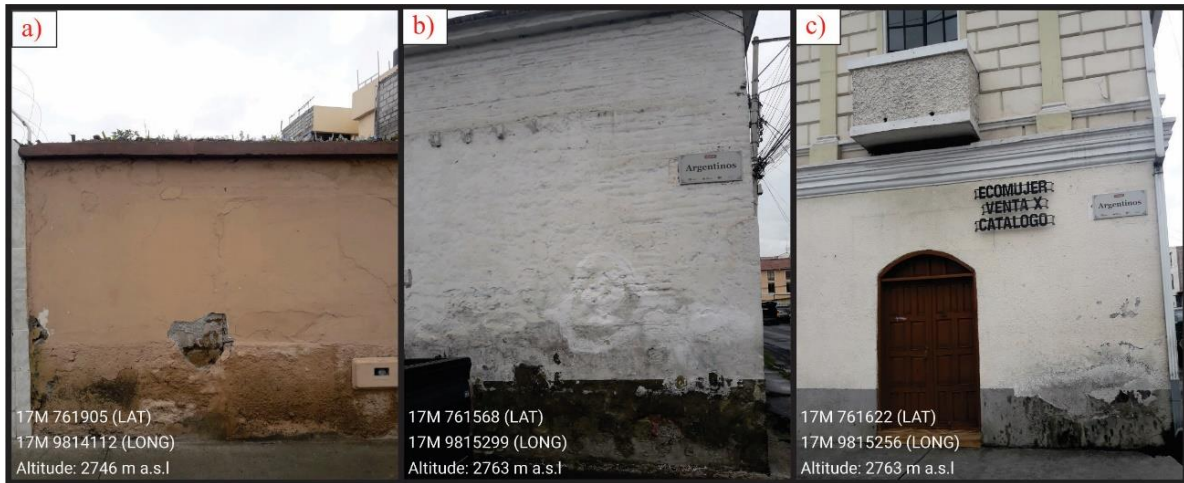
Figure 13. Historical Heritage Buildings of Riobamba City. The figure shows three different kind of historical heritage buildings which were covered or fixed by modern mortar. In these three buildings the salt growing process is limited to the zones covered by modern mortars. The picture a) shows a big hole where the mortar has been removed exposing the rammed earth, inside the wall, to the environment. In the picture b) the deterioration is associated at the mortar surrounding the volcanic rocks arranged in the base of the wall. Finally, picture c) shows slat growing affection in the façade of the building (Author).
