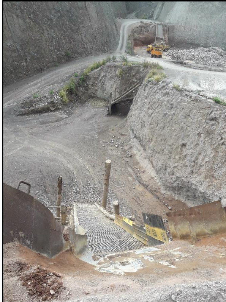
Figure 8. Mira Flores Quarry. The figure shows a typical quarry in Riobamba city. This quarry corresponds to Mira Flores and it is located at the north of the city in the Panamericana E-35 highway. In the background of the image, it is possible to see how heavy machinery mined the material from the deposit. This material posteriorly is sifted to be expended at the citizens (Author).
