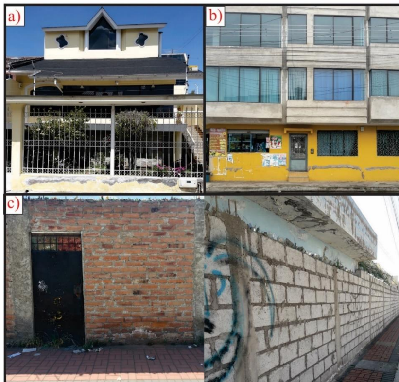
Figure 4. Republican Buildings in Riobamba city. The figure shows the typical republican buildings and its classification according to the ending of the building. a) shows a typical republican building built in base of concrete, bricks, iron, and aggregates. Likewise, a) is a white work building because the walls are cover by a white plaster and painted b) this picture shows a building where the ground floor corresponds a white work. However, the upper floors are designed as gray work building due to, the endings correspond a wall cover by mortar without protection against the environment. Finally, both walls showed in c) there are two different black work building because bricks (terracotta, concrete) and columns does not have any protection (mortar, paint) against the environment (Author).
