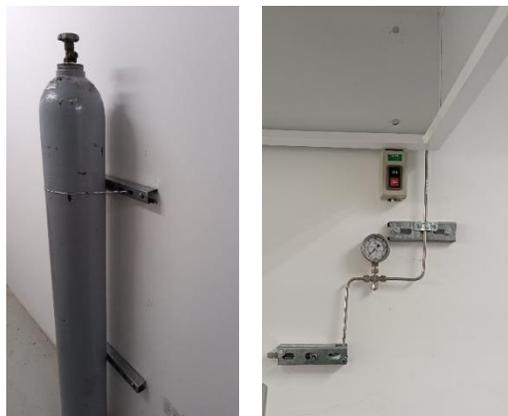
*Figure 25. CO<sub>2</sub> Feeding system*
